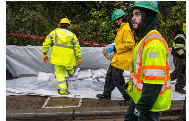
Members of the San José Conservation Corps pile sandbags along the San Francisquito Creek in East Palo Alto on Jan. 4, 2023. The creek spilled over its bank and into a nearby community during the storm on Dec. 31. (Beth LaBerge/KQED)
