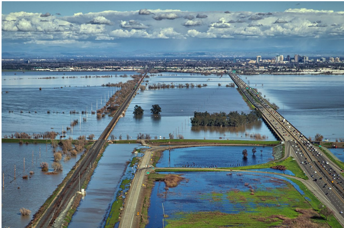
Yolo Bypass (Sacramento River Flood Control Project) 1917
