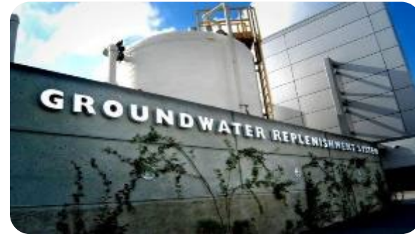
RO-treated Recycled Water
