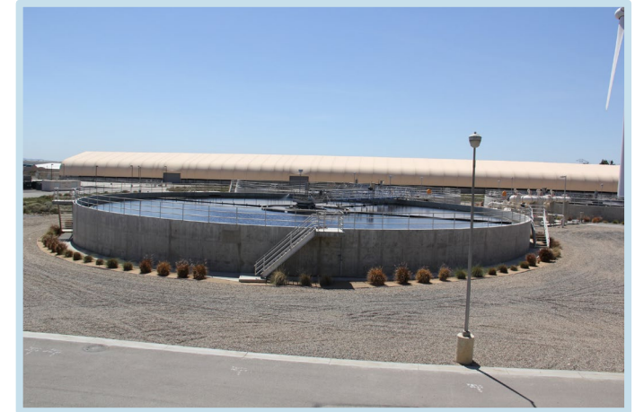
IEUA's Regional Water Recycling Plant No. 4 in Rancho Cucamonga.
