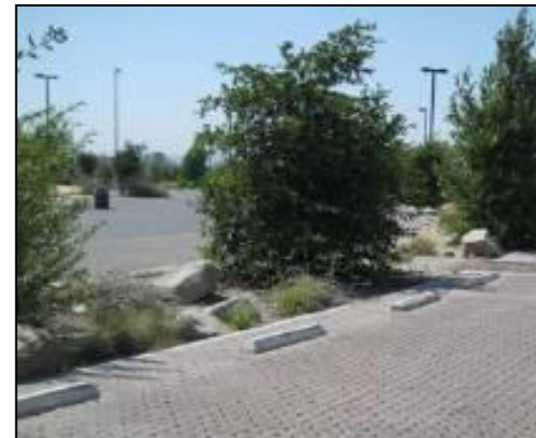
Porous Pavement – Rio del Los Angeles State Park (aka: Taylor Yard)
